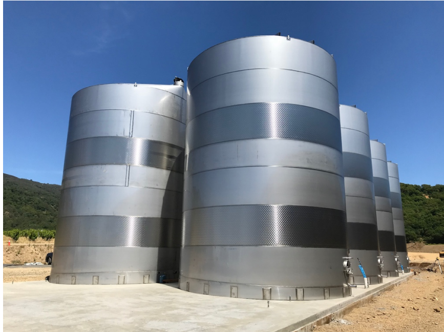
Figure 2: Liquid storage tanks built according to the tank construction drawings
